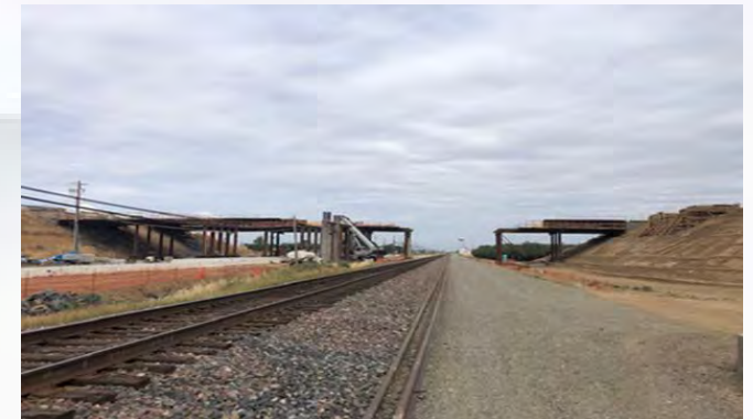
Campus Parkway Segment II, spanning Hwy 140 (May 15th, 2019)
